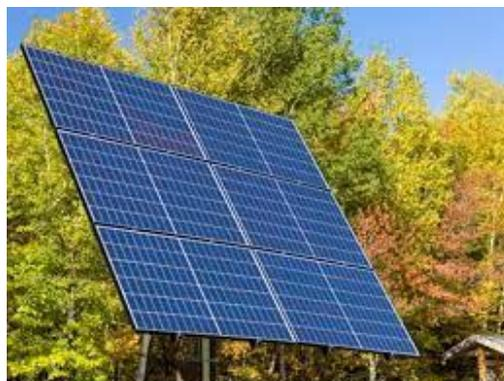
Passivated Emitter and Rear Cell type of solar panels are an improved version of the traditional monocrystalline cell. This technology employs the addition of a passivation layer in the cell's rear surface and hence the efficiency is improved. Light is reflected back into the cell and hence
