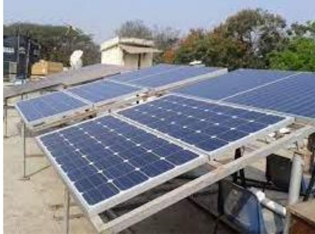
Polycrystalline panels are produced from more than one silicon crystal. The fragments of silicon are melted and poured into a mold. Hence the cost of polycrystalline panels is less and affordable. However such panels are less efficient in converting solar energy and occupy more space. These panels exhibit lesser heat tolerance that is they perform poorly in environments of high temperature.
