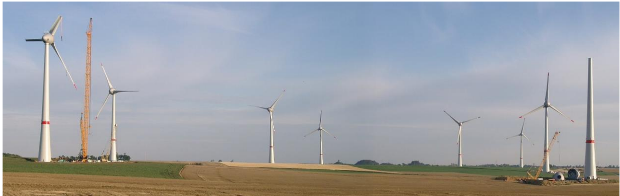
Fig. 5 First wind farm consisting of 7.5 megawatt (MW) Enercon E-126 turbines, Estinnes, Belgium, 20 July 2010, two months before completion.
