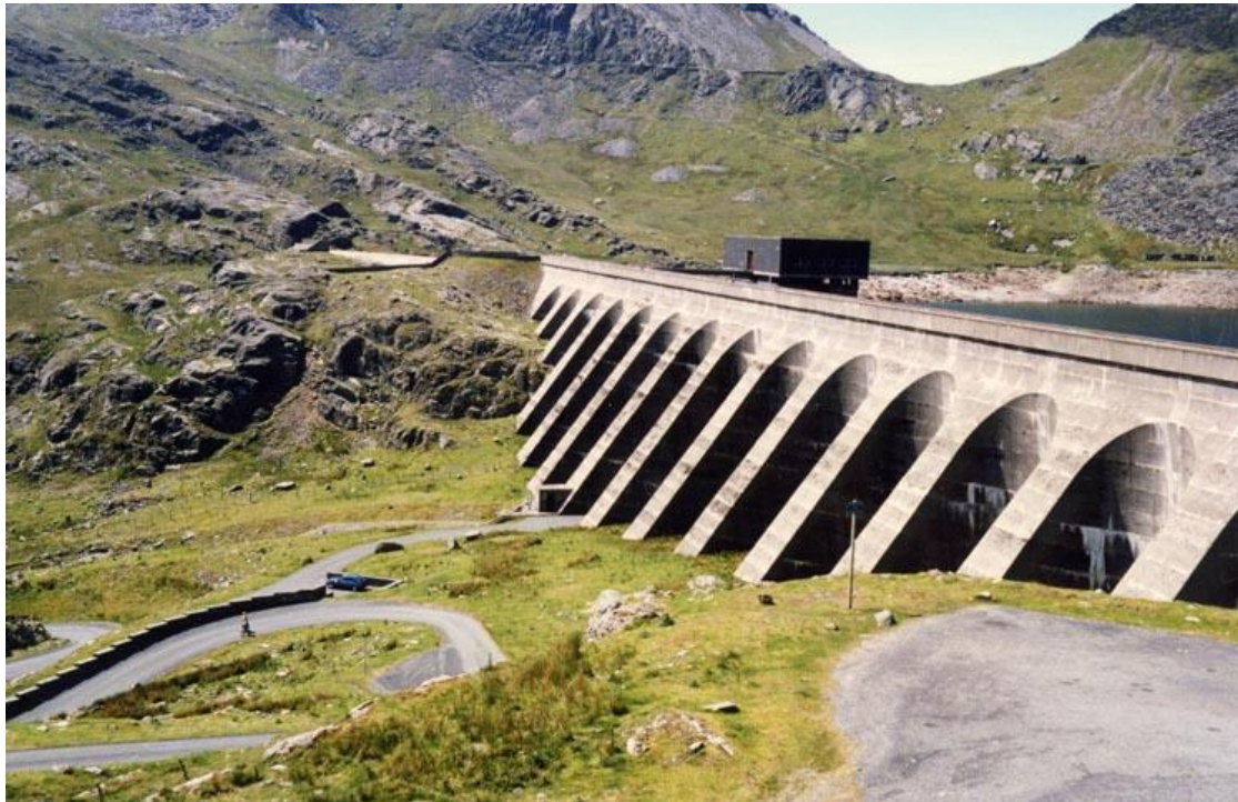
Fig. 15 Pumped-storage hydroelectricity – the upper reservoir (Llyn Stwlan) and dam of the Ffestiniog Pumped Storage Scheme in north Wales. The lower power station has four water turbines which generate 360 MW of electricity within 60 seconds of the need arising
