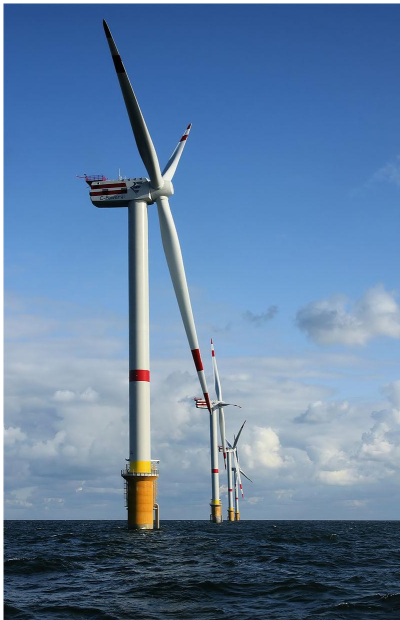
Fig. 6 Offshore wind farm, using 5 MW turbines REpower 5M in the North Sea off the coast of Belgium.
